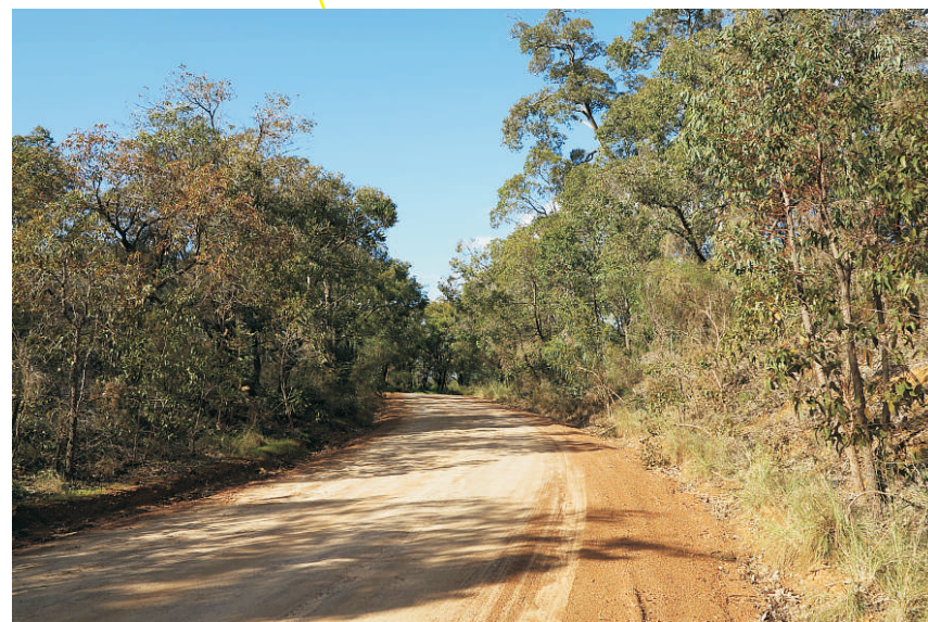
Pruden Road, view east
