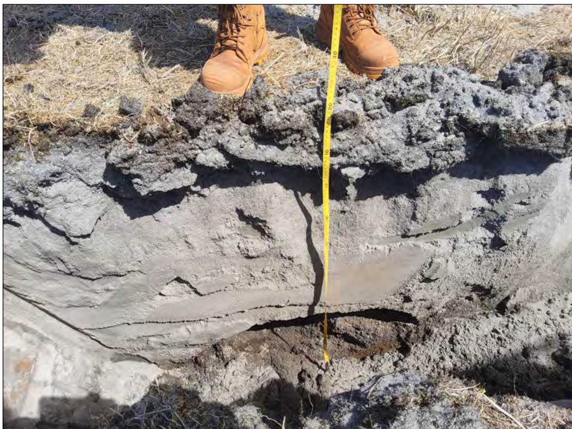
TP10: Downhole view
