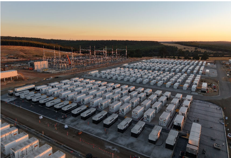
Figure 5: SynergyRED owned 500MW Collie Battery Energy Storage System (under construction)
