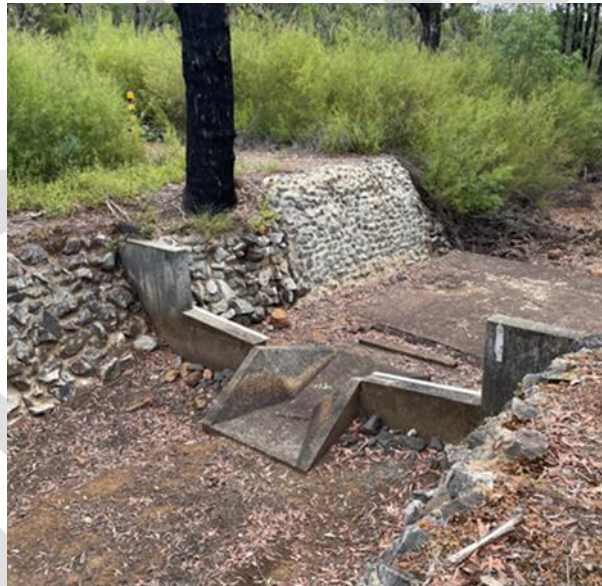
Figure 4.2: Typical Small-Scale Streamflow Gauging Structure
