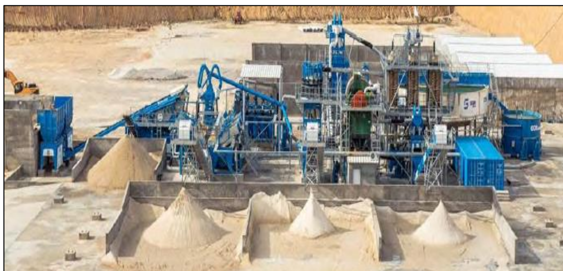
Plate 2-3 Example Image of a Typical Sand Processing Plant
