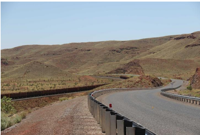
Plate 25: Enclosed north view from Manuwarra Red Dog Highway (view location 23)
