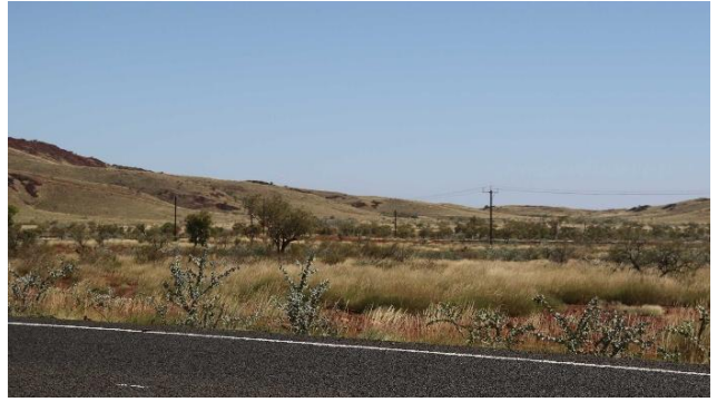
Plate 4: Transmission line at view point 34
