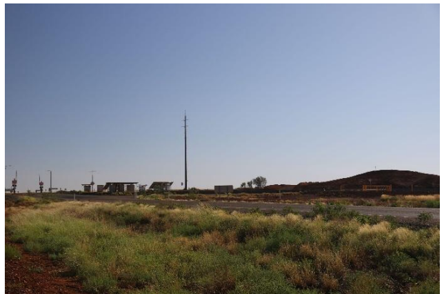
Plate 8: Rail Crossing (view point 13)
