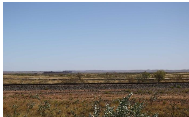
Plate 2: Pipeline and rail at view point 33
