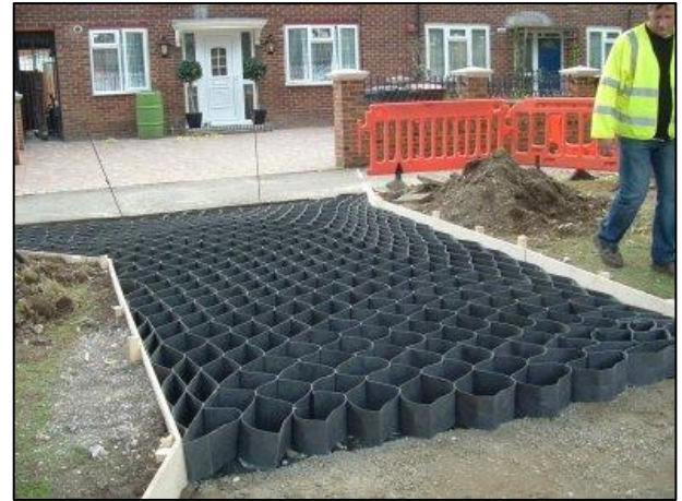
Image 4 – no dig pathway installed over tree roots Image 5 – Geocells pre instalment of trafficable material
