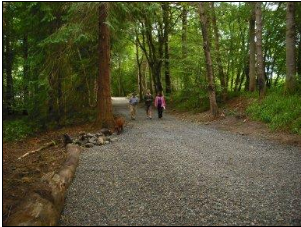
Image 4 – no dig pathway installed over tree roots Image 5 – Geocells pre instalment of trafficable material
