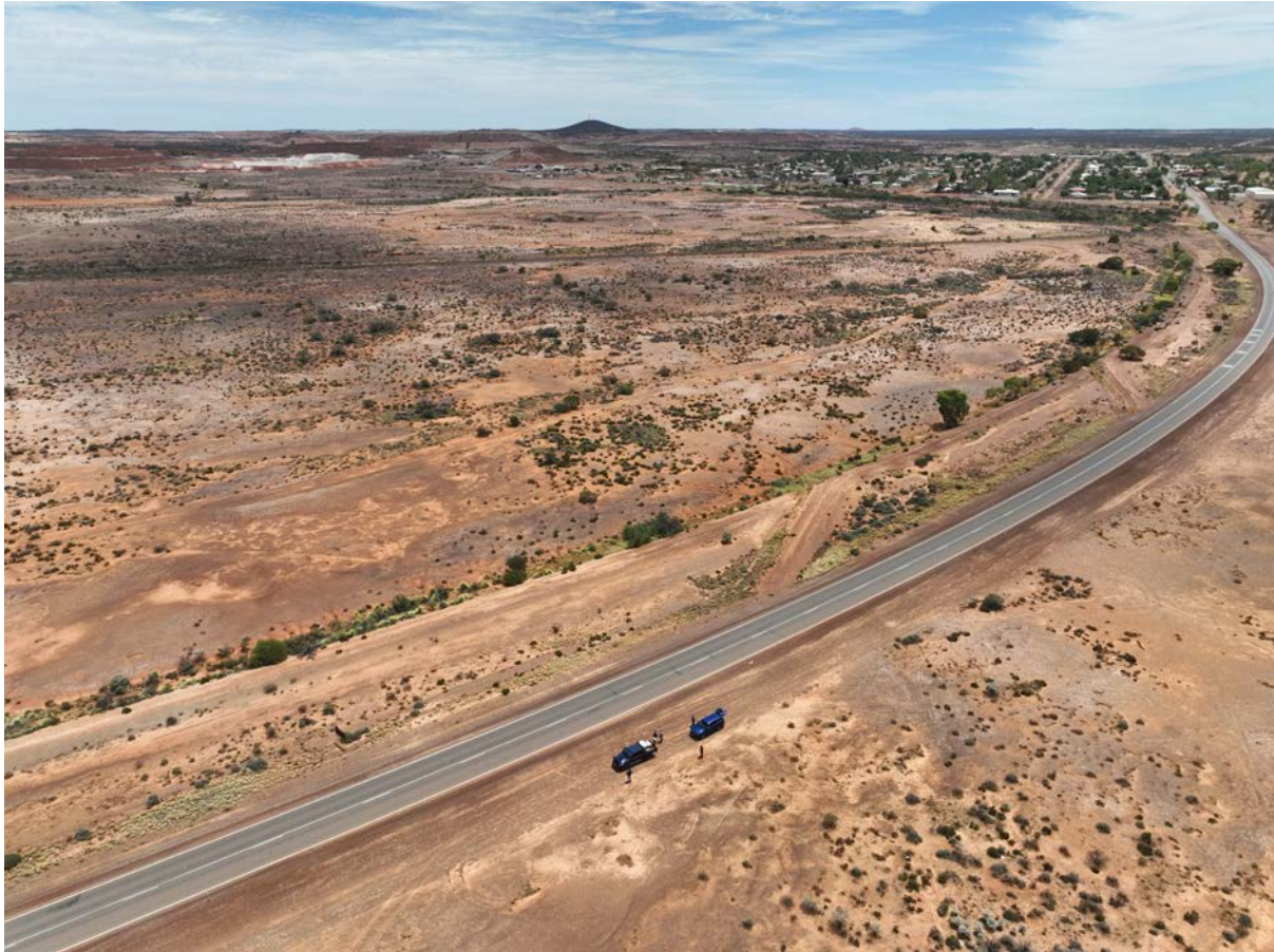
Image 12: Looking west towards the new Mt Magnet blade bypass
