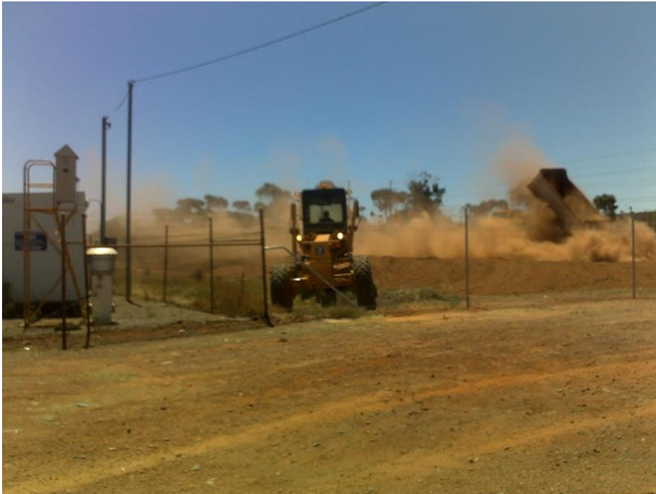
Figure 9: Non-KCGM Related Earthworks at BSY PM 10 Monitoring Site – October 2012
