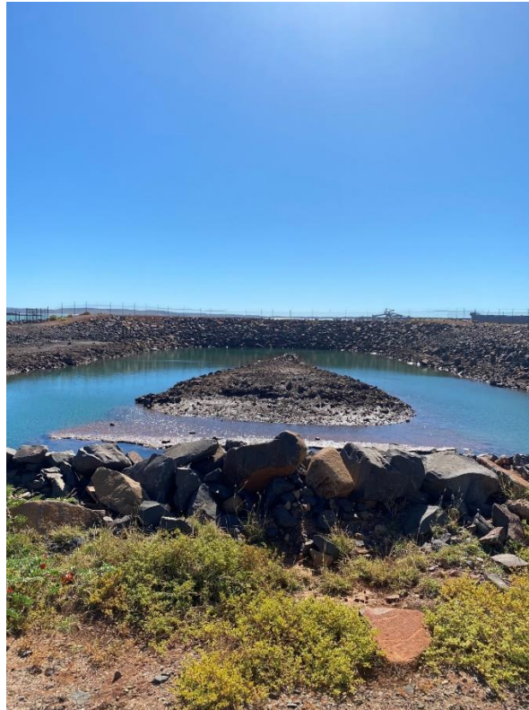
Figure 1: Existing intake pond
