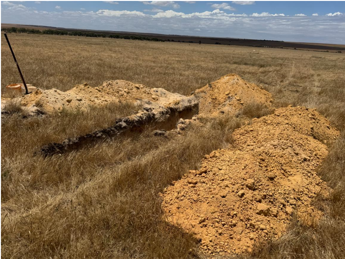
Figure 8: Material excavated from Test Pit 4.
