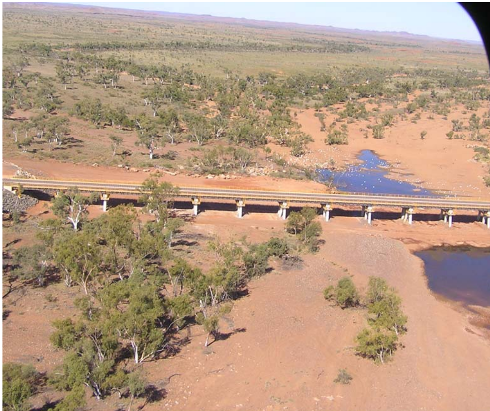
Figure 5 BHP rail crossing Yule River
