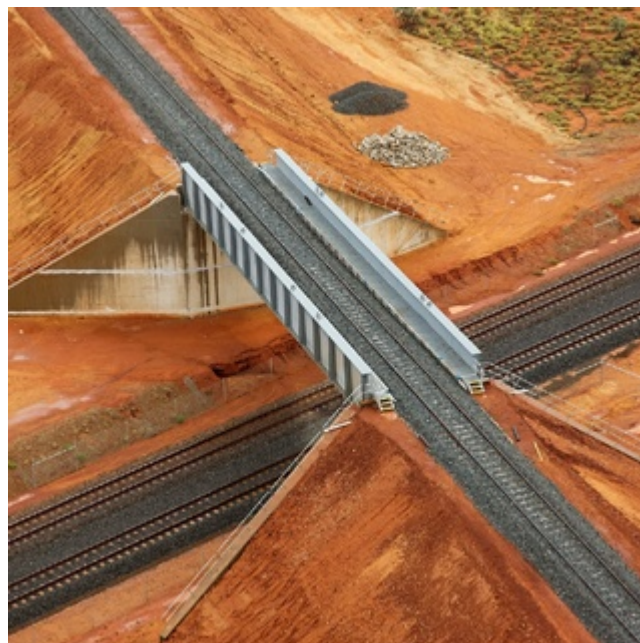
Figure 7 FMG bridge crossing BHP line
