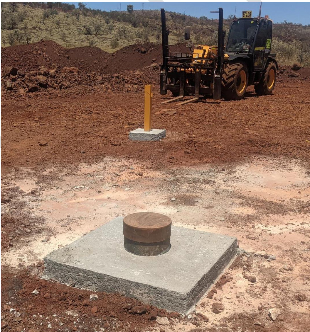
Figure 5: HMN0042-P and HMN0046-M headworks
