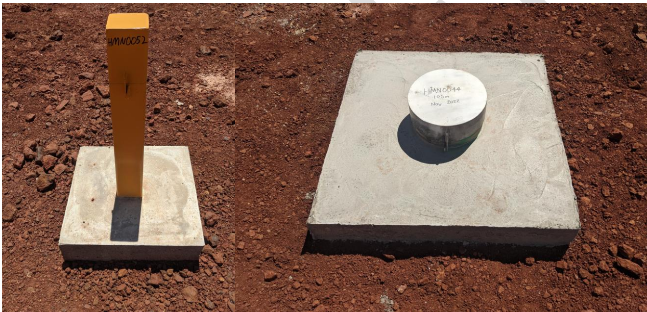
Figure 4. Monitoring bore completion (Left) Production bore completion (Right)
