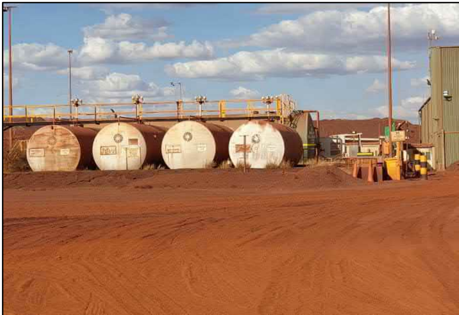
Photograph 8: Fuel farm with ASTs
