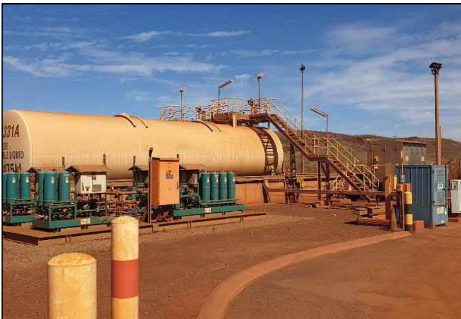
Photograph 11: Fuel farm with ASTs
