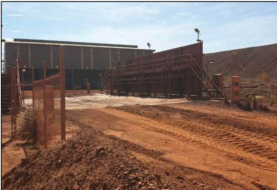
Photograph 12: Mining plant and equipment washdown area
