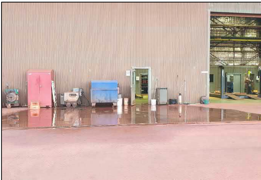
Photograph 7: Equipment cleaning area at the Infrastructure – OHP Maintenance Workshop
