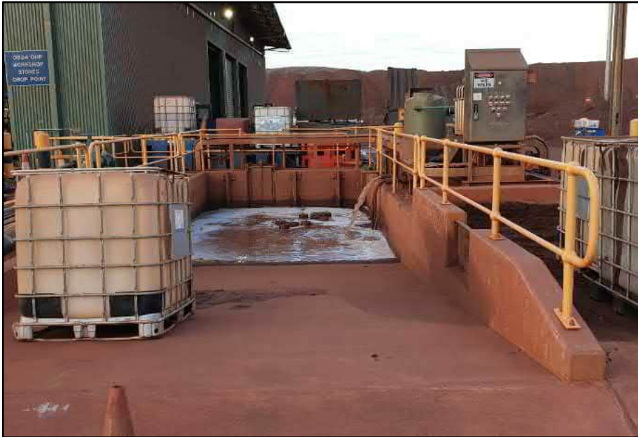
Photograph 6: Water processing system in front of OB24 OHP Workshop stores drop point
