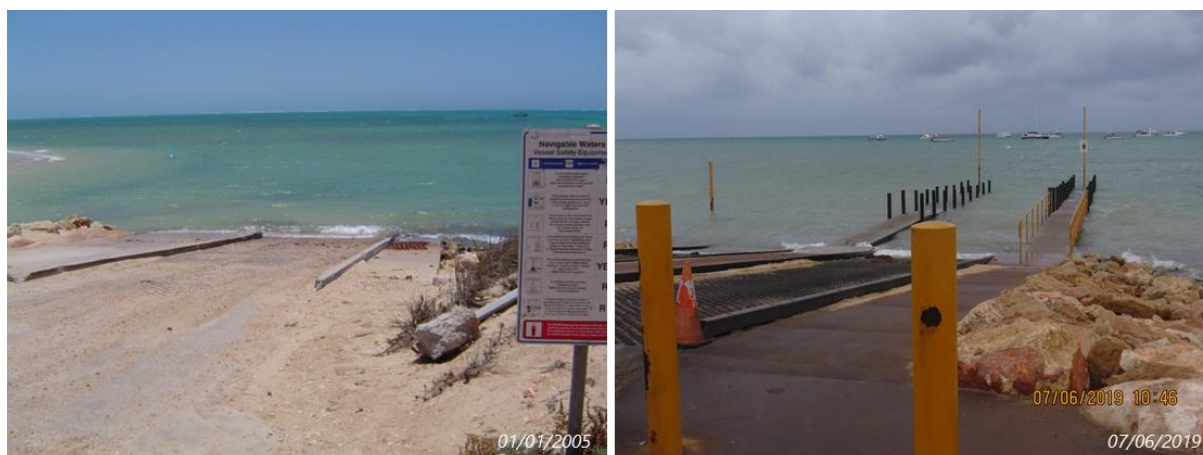
Plate 2. Tantabiddi Boat Ramp upgrades. Left: the single lane boat ramp pictured in 2005. Right: the ramp was upgraded in 2012 to a dual ramp with two finger jetties (photo captured 2019).
