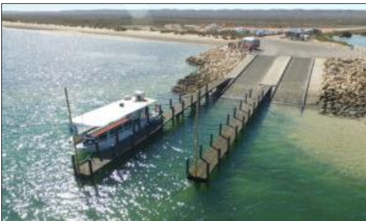
Plate 17. Top: the estuarine sand bar accumulates on the southern side of the boat ramp and reduces the depths for boat access (Photo: West Regional/Branwen). Bottom: view looking north east shows the relative lack of sand accumulation on the northern side of the ramp (Photo: Ningaloo Ecology Cruises).
