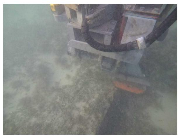
Figure 5 Subsea rig setting up at BH03 – timber protecting seabed visible below mast plate
