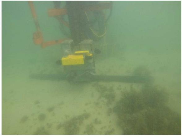
Figure 6 Mast erected at position of BH13 in advance of drilling
