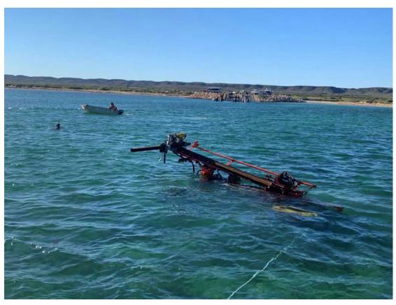
Figure 1 Subsea rig tracking from BH04 to BH08 immediately NW of existing boat ramp. Snorkeller and TAMS tender in attendance to safeguard passing boat traffic
