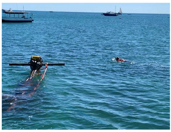
Figure 3 Subsea rig tracking underway from BH08 to BH10 within boat mooring area
