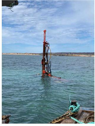
Figure 2 Subsea rig set up at position of BH13
