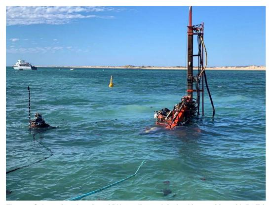
Figure 1 Subsea rig at location of BH04 – diver at left checking position with R1 Trimble GPS unit visible on pole
