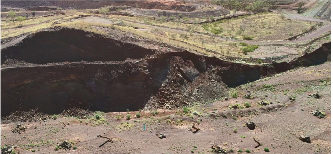
Figure 5-110 E1 diversion oblique view example of erosion / slumping
