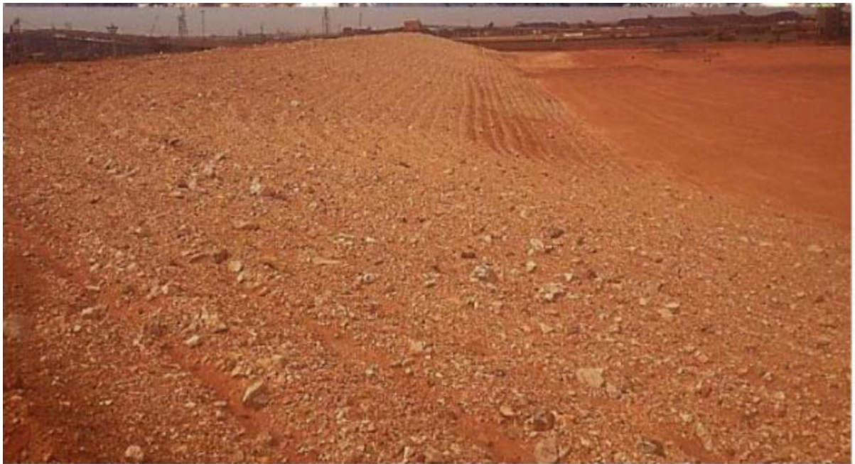
Figure 9-9 Contour ripping
