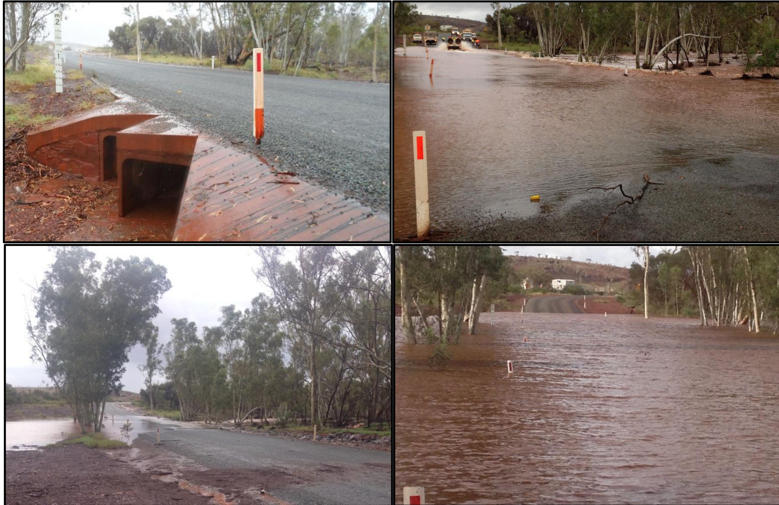
Figure B-32. Homestead Creek at Marble Bar Road Floodway 21-22 January 2014
