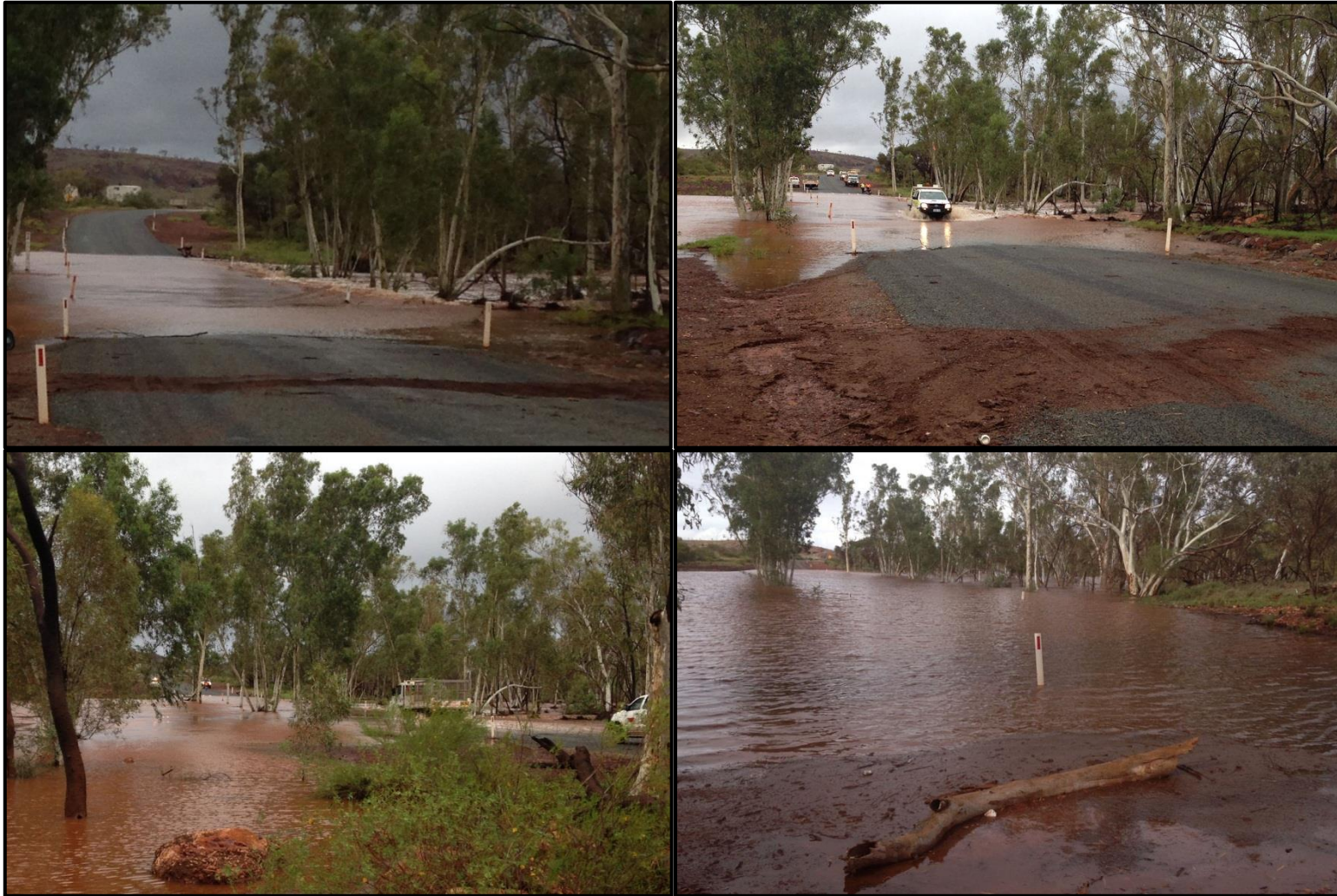
Figure B-33. Homestead Creek at Marble Bar Road Floodway 21-22 January 2014
