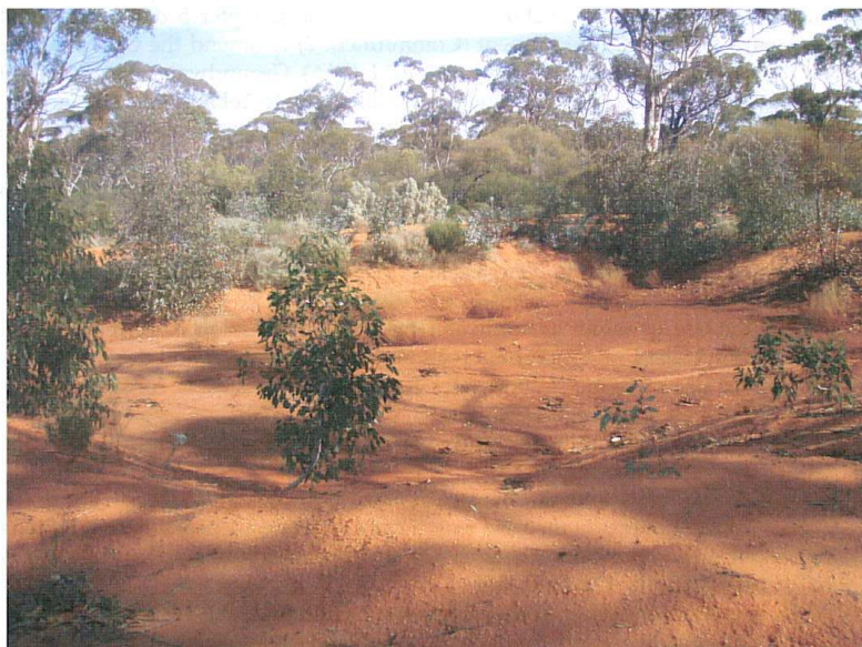
Figure 2. Photograph of a road sump on the Haul Road. Sumps occur along the length of the Haul Road to contain road runoff. Road runoff is directed to the sumps by the road grading and bunding. (Photograph: S Hawkins, May 2008).
