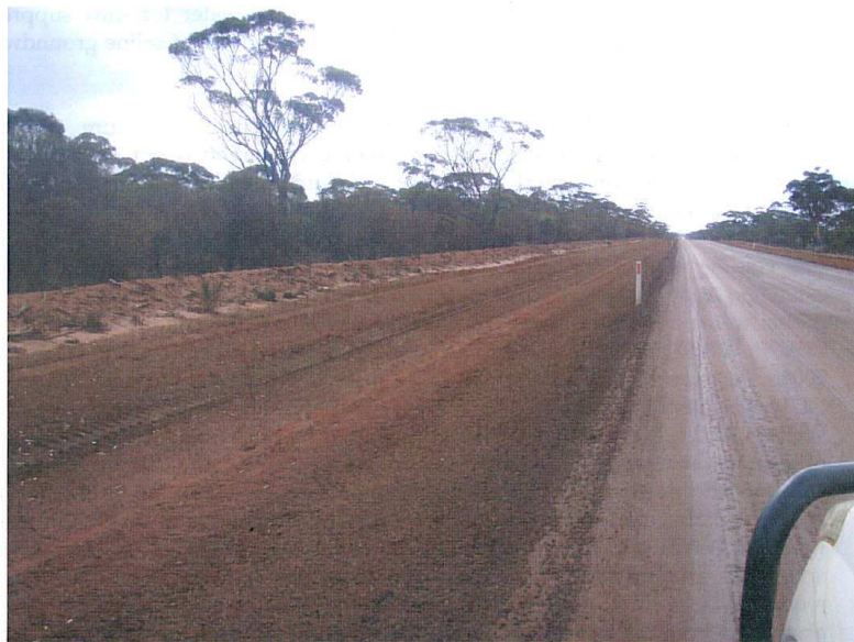
Figure 1. Photograph of road drainage and bunding on the Haul Road. The Haul Road is graded and bunded to ensure that saline groundwater used in dust suppression does not escape into the adjacent native vegetation. (Photograph: S Hawkins, May 2008).
