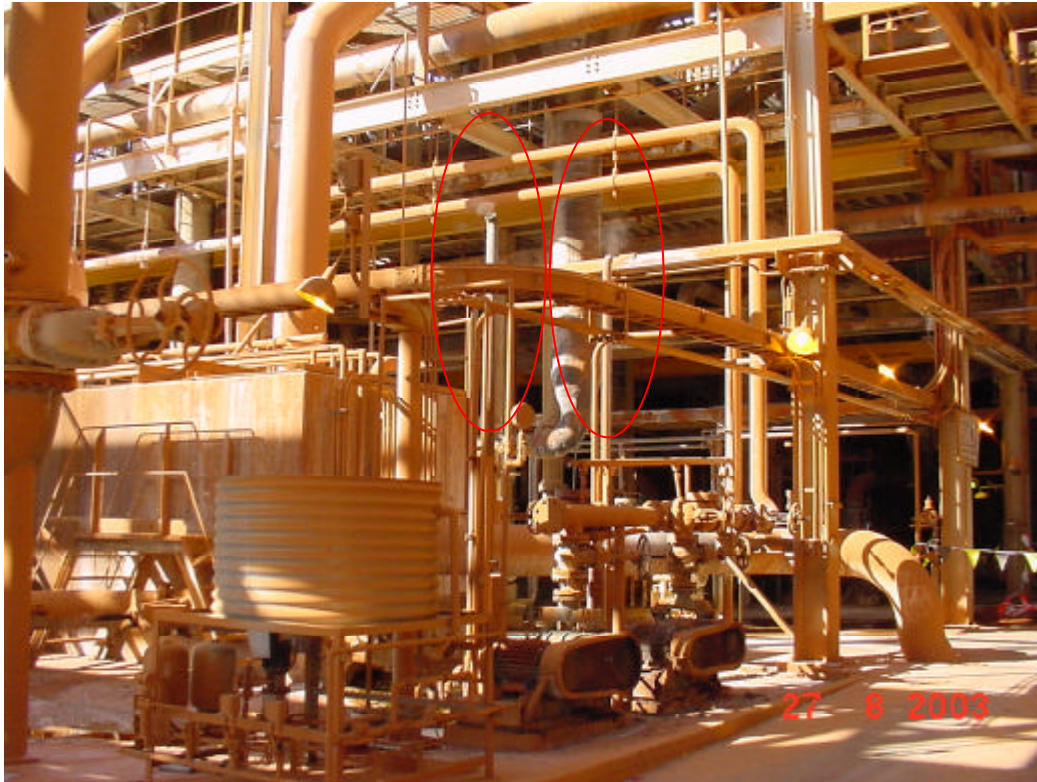
■ Figure 27 Building 42, 3 & 4 Vacuum Pump Vents
