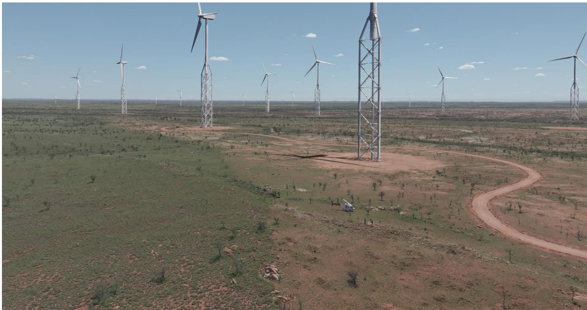
Plate 3-3 Access roads to the wind turbines
