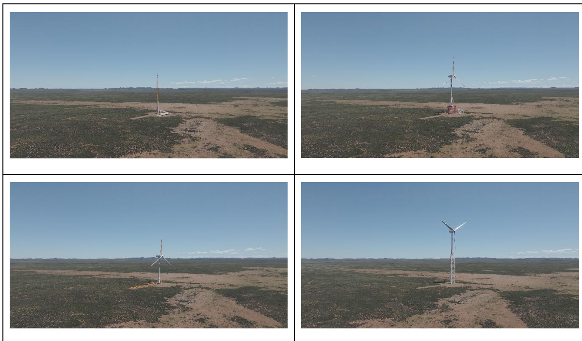
Plate 3-1 Nabralift Tower Construction
