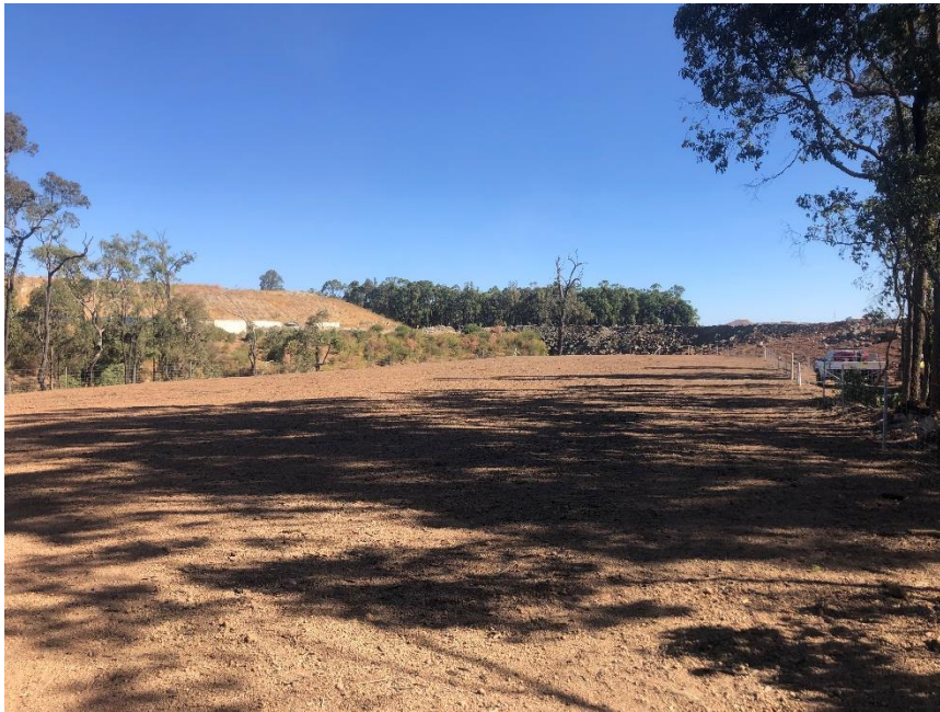
Figure 5: MSA WWTP Spray Field Clearing Area
