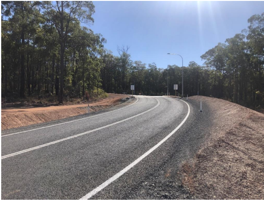
Figure 3: Stanifer Road Access Clearing Area
