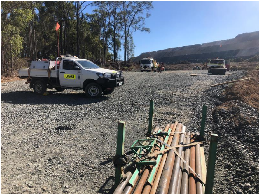
Figure 4: Drillers Laydown Area Clearing Area
