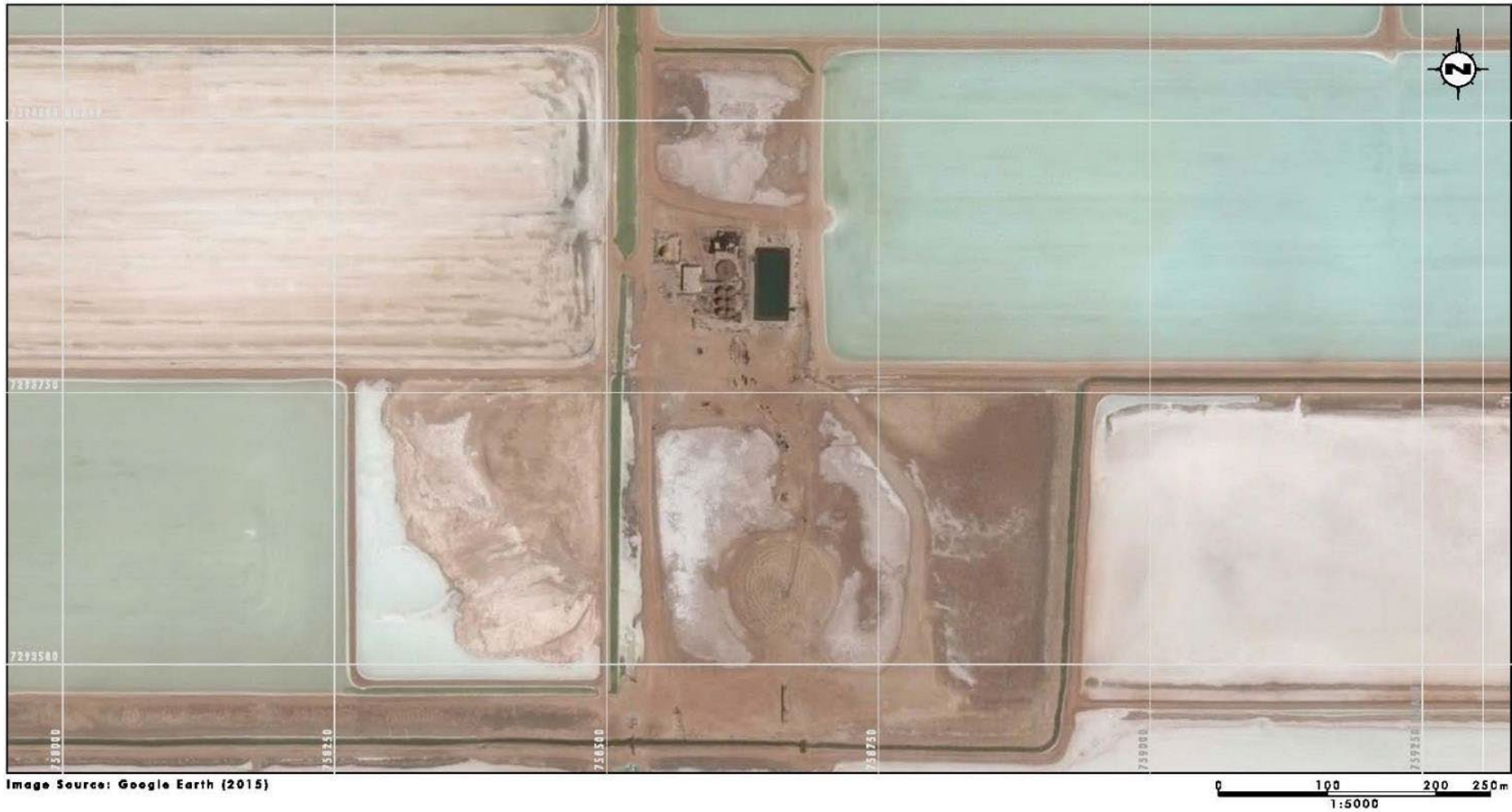
Decommissioned Potash Production Facility
