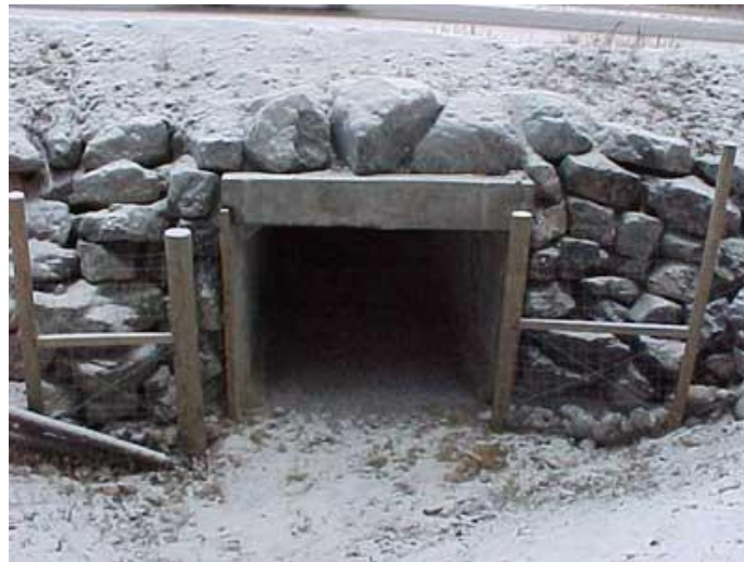
Figure 2: Example of a typical box culvert used in North America to help facilitate small animal movement under a busy road. (Sourced: Parks Canada).
