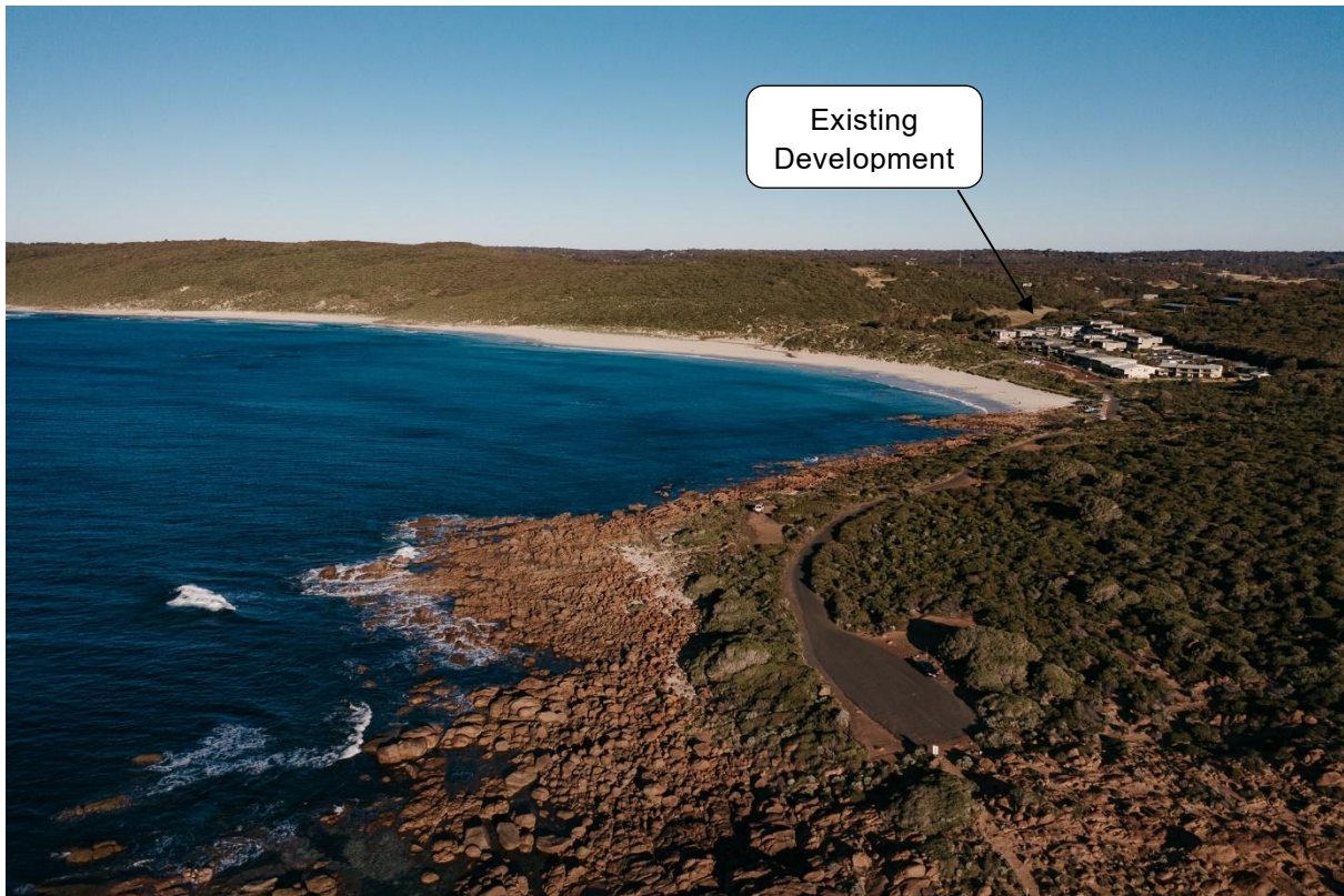
Figure 1.3 Smiths Beach Looking East
