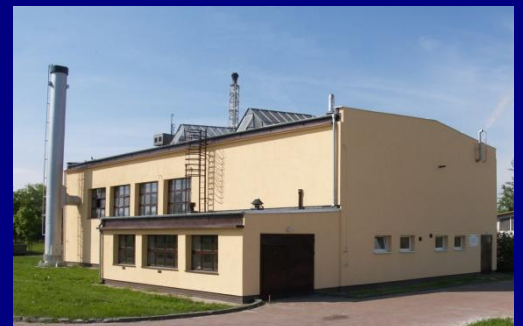
→ WtGas Plant Building
