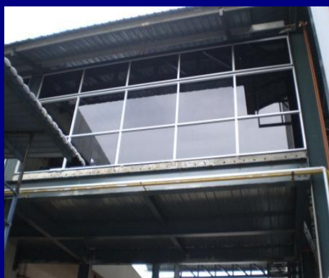
← Plant Control Room
