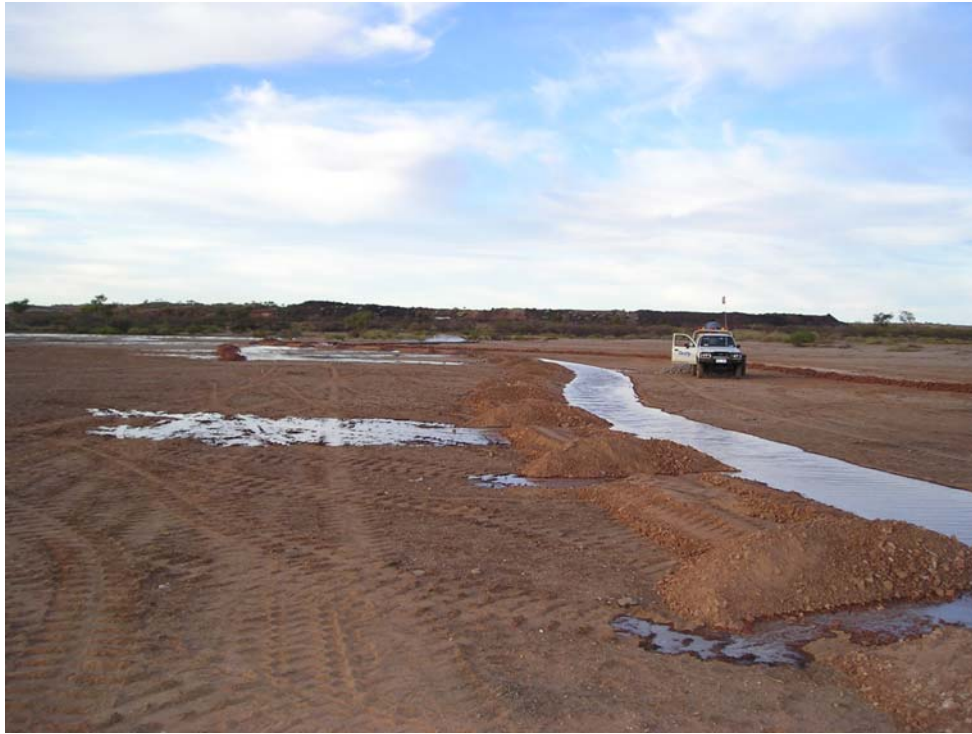
Picture 8: Preferential flow from spreader ditch.
