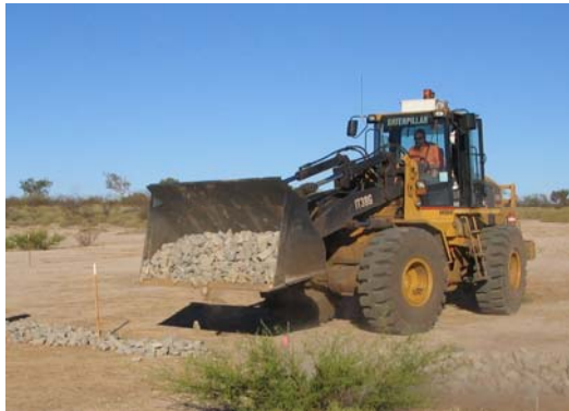
Picture 1: Constructing trial levees
