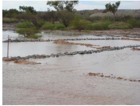
Picture 14: Peak capacity of 40 m of levee at 170 l/sec discharge
