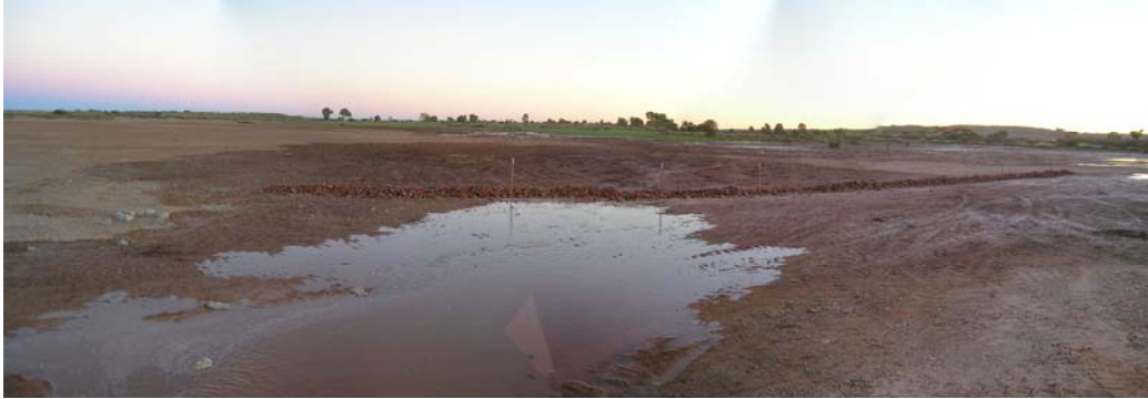
Picture 11: Levee across undulations, start day 2. Initial flow from gaps in the spreader ditch has been channelled in the depression, until it reaches the wall. The dark areas show the extent of back-up and sheet flow from the previous day's trial.
