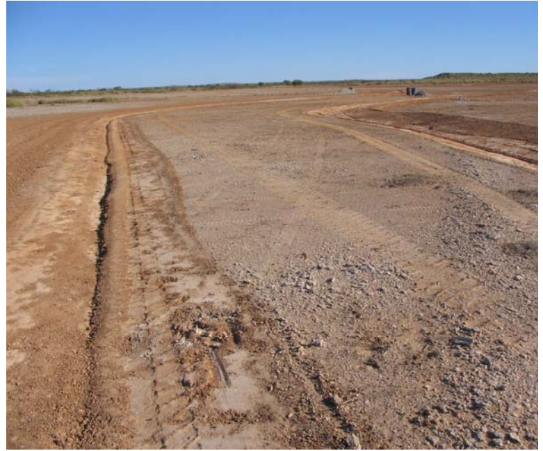
Picture 5: Spreader ditches: lower side undisturbed on upper ditch, and spoil on downslope side on lower ditch.
