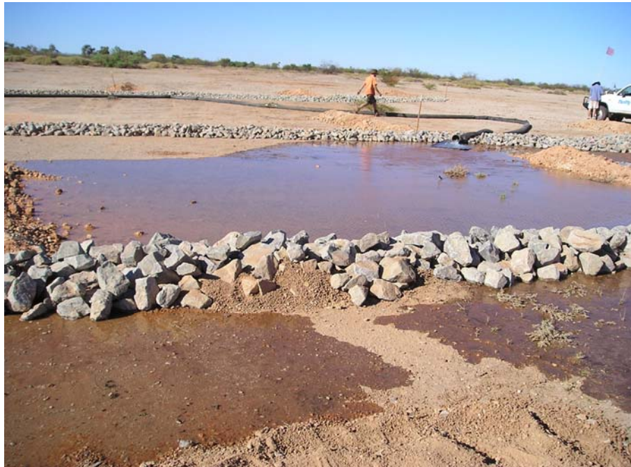
Picture 4: Fines mixed with screened rock prevent flow.
