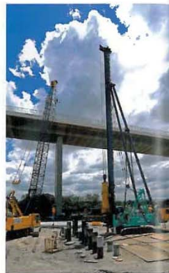
Driving piles for the approach pier.
