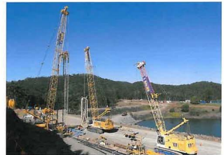
Bauer is installing the cut-off wall at the Hinze Dam expansion.
