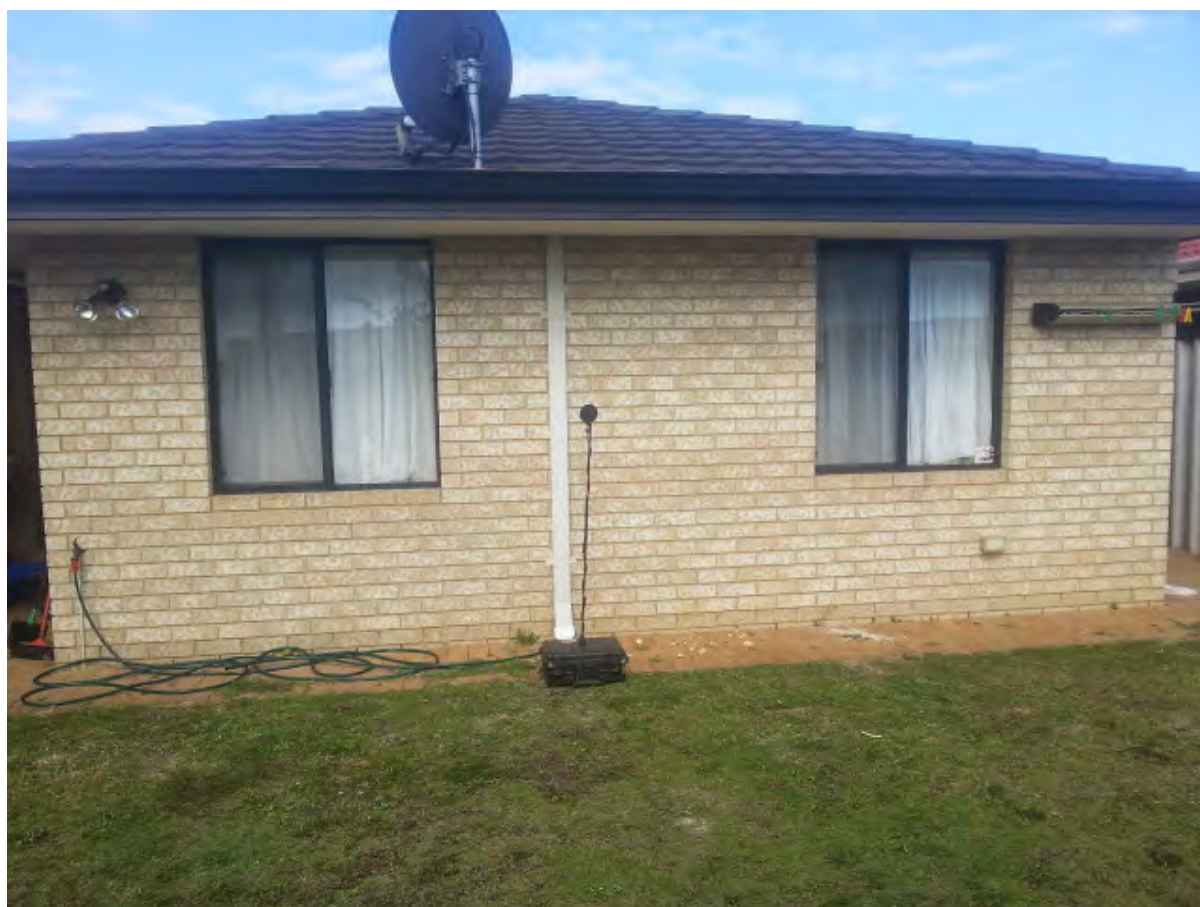
Photograph A13– Noise Logger at 43 Mitra Loop, Beechboro
