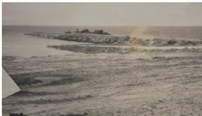
Plate 6: Reconstruction works, rockfill and barge hardstand (NAA)
