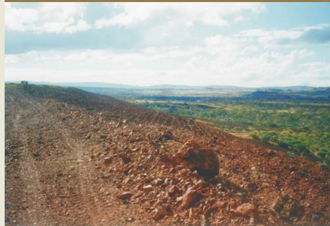
Final Batter Not Greater than 20°
