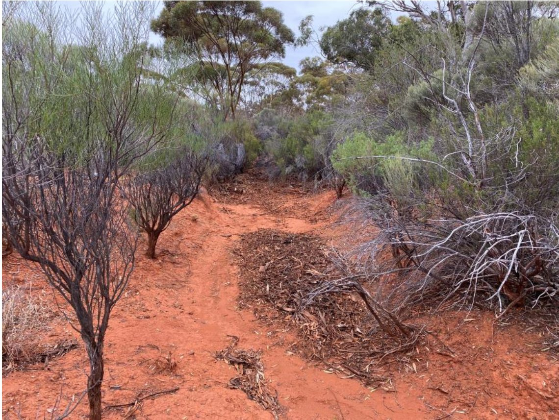
Plate 2-3: Small break in earth bund allowing combination of flow
