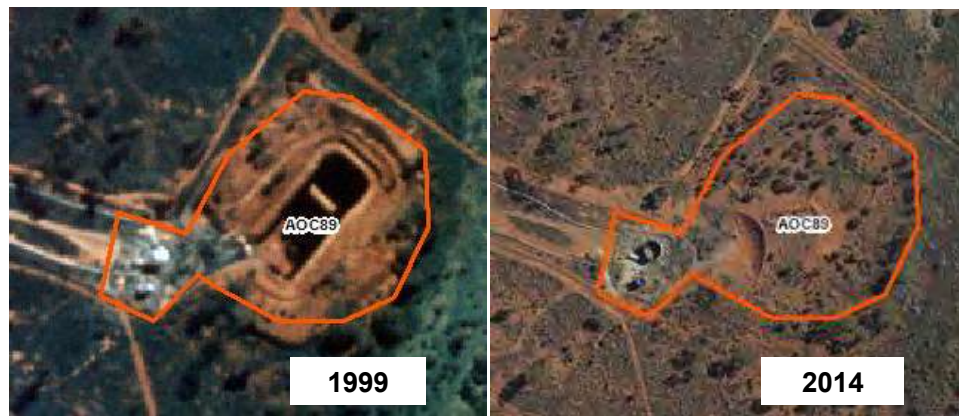
Figure A18: AOC89 Saline water transfer station
