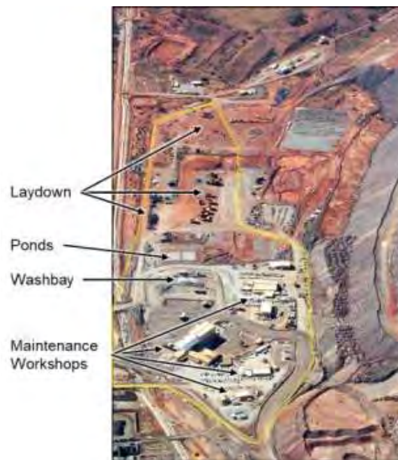
Figure 9: Contractor Workshops 2017 (facing east)
