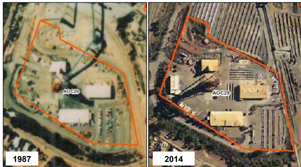
Figure A11: AOC 29 – Workshops and hydrocarbon storage area at the Cassidy headframe
