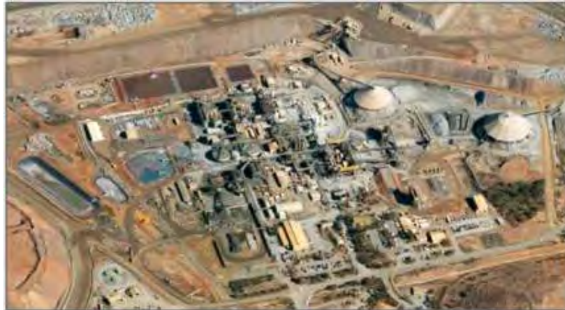
Figure 8: Fimiston Mill 2017 (facing west)
