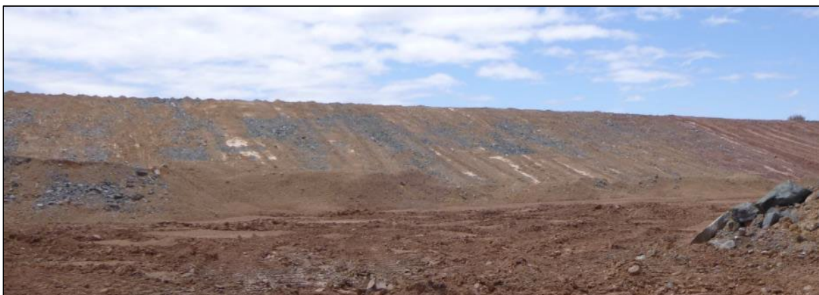
Figure 5-35: OTD Remedial Works in Progress 2017 (Oroya WRD)
