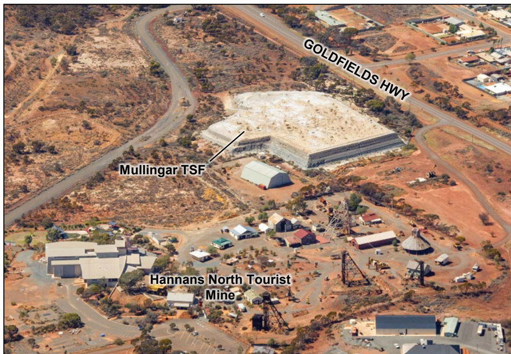
Figure 5-106: Mullingar Tailings Storage Facility (2021)
