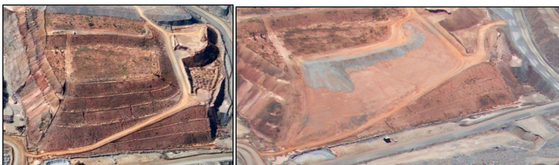
Figure 5-33: Radio Hill Prior to 2017 (Left) and during 2017 Remedial Works (Right)
