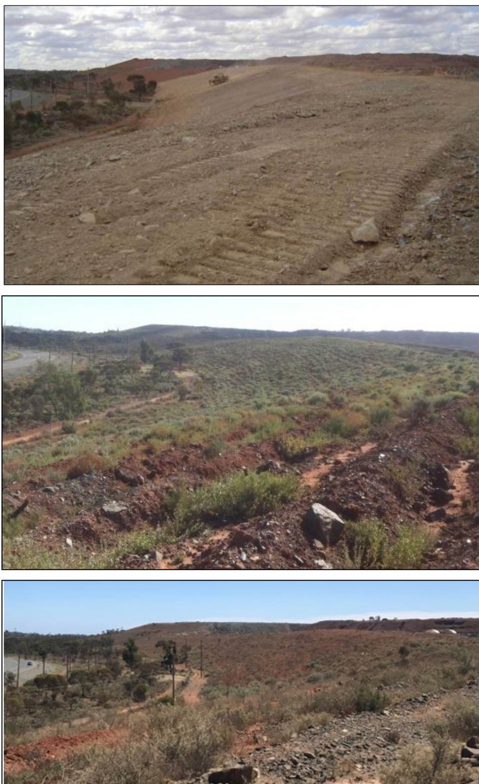
(Top: Battering 2011. Middle: 2013 Progress of rehabilitation Bottom: 2021)
