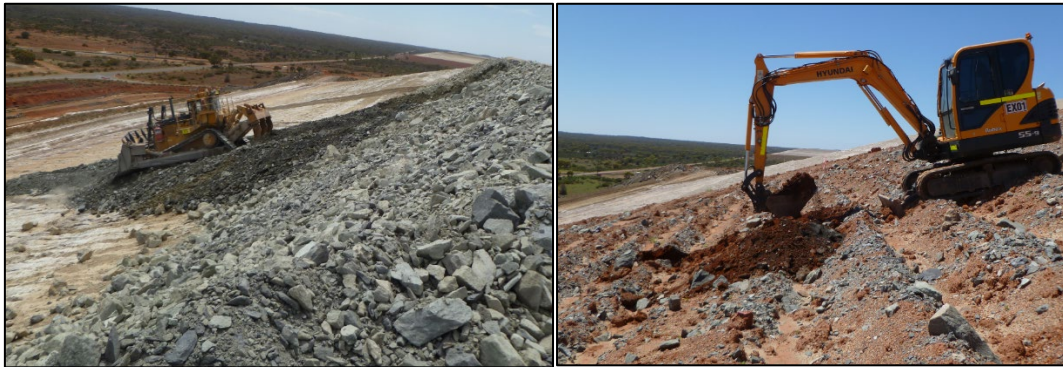
Figure 5-60: Fimiston I TSF Trial Earthworks in Progress (2016 and 2017)
