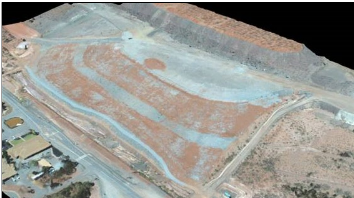
Figure 5-43: Old Croesus 2021 Capping and Completed Rehabilitation
