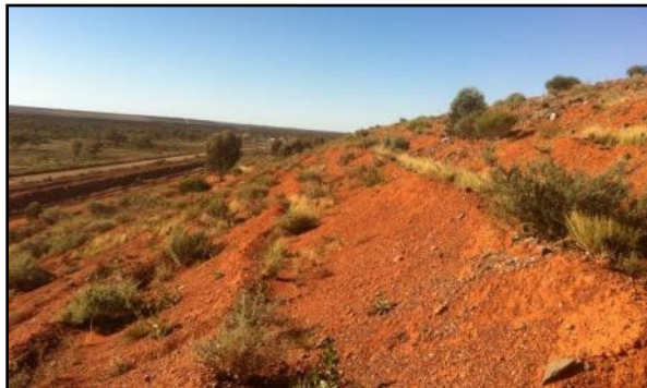
Figure 5-59: Typical Fimiston I TSF Batter (2013)
