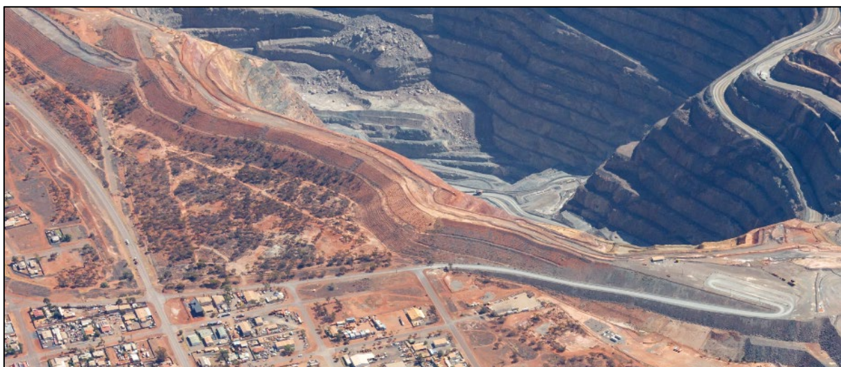
Figure 5-49: Southern Noise Bund (2021)
