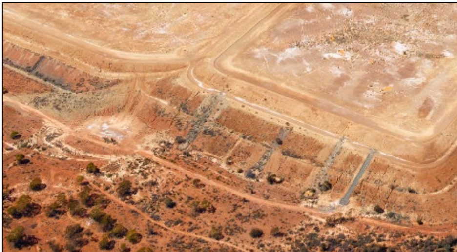
Figure 5-103: Erosion and Water Control Repairs on Mt Percy TSF Completed in 2019 (2021)
