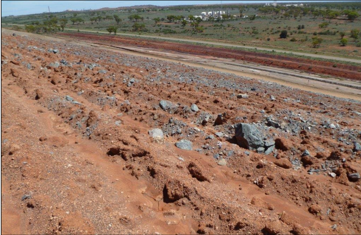
Figure 5-110: Fimiston I TSF Trial Immediately after Completion of Earthworks (Feb 2017)
