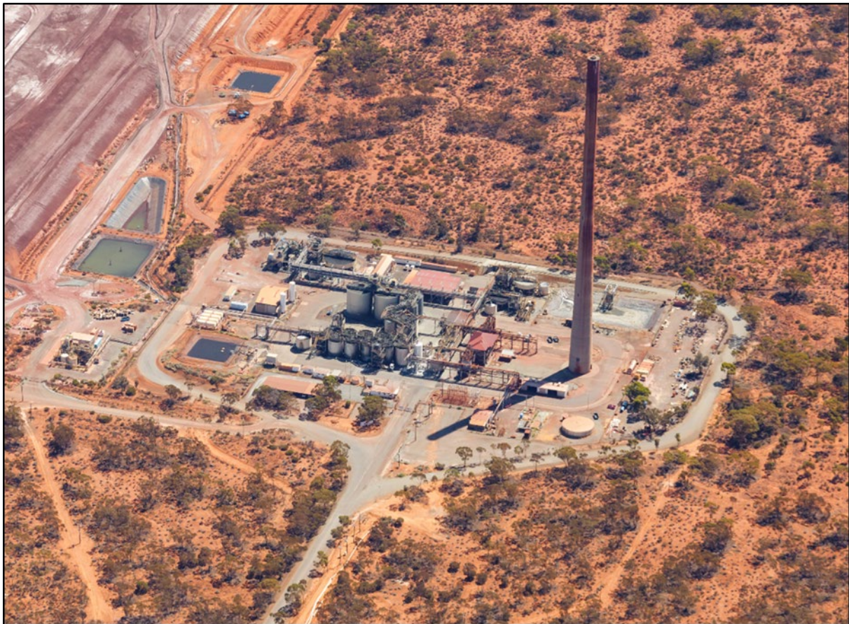
Figure 5-81: Gidji Processing Plant (2021)
