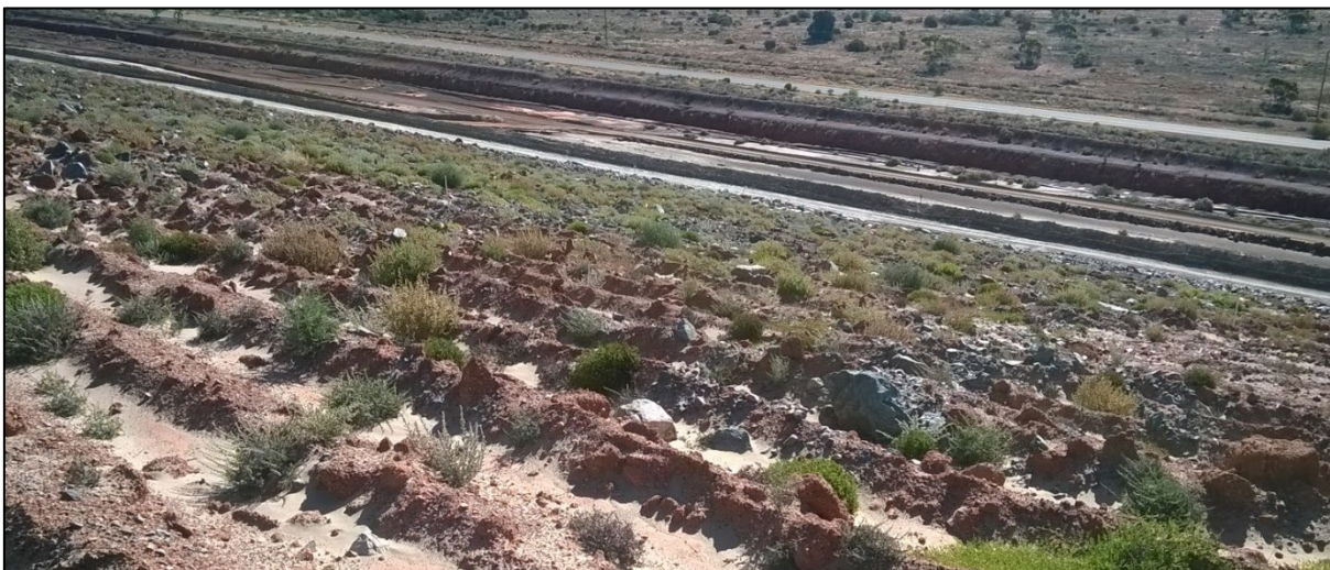
Figure 5-111: Fimiston I TSF Trial Observed Germination after Rains (July 2017)
