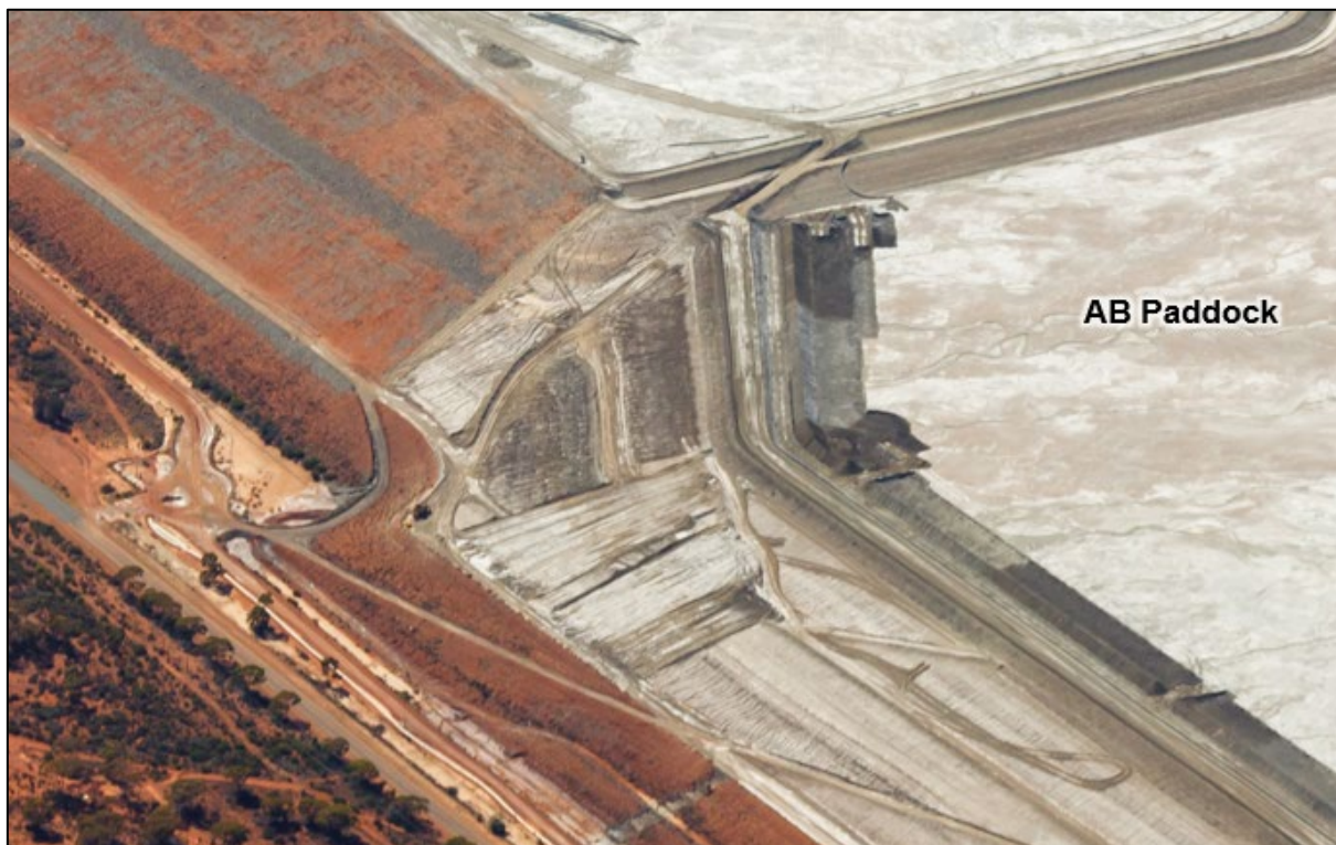
Figure 5-70: Fimiston II TSF 2021 commencement of reshaping of AB Paddock
