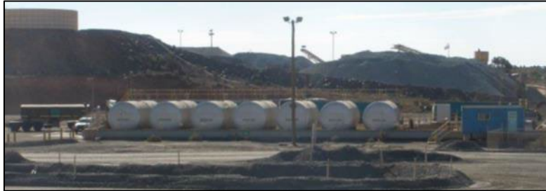
Figure 5-20: Fimiston Mining Fuel Farm
