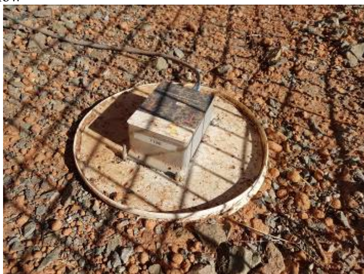
Figure 3.2: Typical Vibration Geophone setup adjacent to the KCGM Fimiston Open Pit
