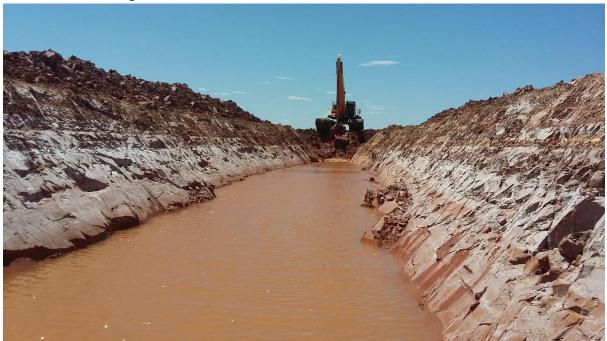
The walls held up reasonably well although areas of collapsing were evident. After 50m the trench was narrowed for a few meters however after some collapsing occurred (and the reduced width) it was decided to keep the wide trench design. The trench length was 100m including ramps on North and South ends. Average width is 13m with the depth based on the required design of 6m.
