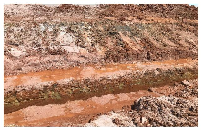
The walls held up well, with no collapses evident. This allows for a consistent trench width and depth for the entire 100m.
