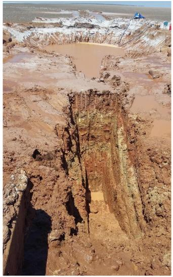
The walls held up reasonably well, most likely due to the occurrence of the hard gypsum sand layering. The trench length was 100m including ramps on North and South ends. Average width is 13m with the depth based on the required design of 6m.
