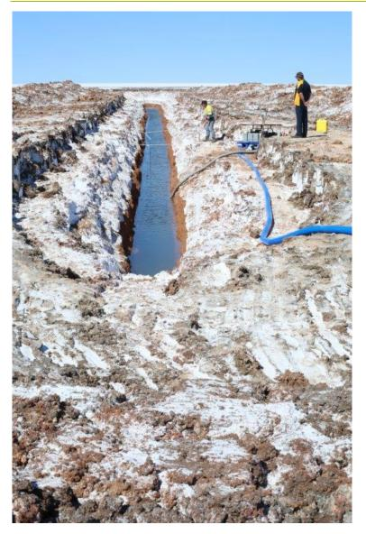
Photograph 3: Groundwater extraction for hydrogeological studies
