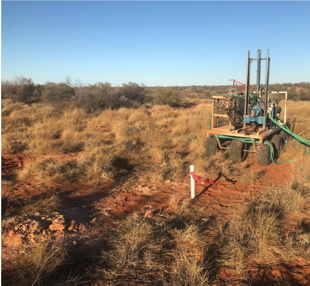
Figure 4. Example of bore installation
