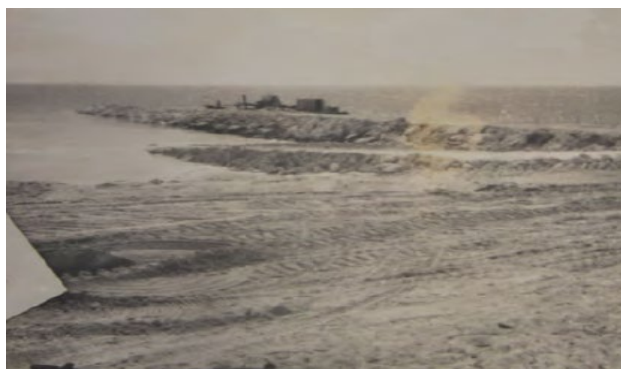
Plate 6 Reconstruction works, rockfill and barge hardstand (NAA)
