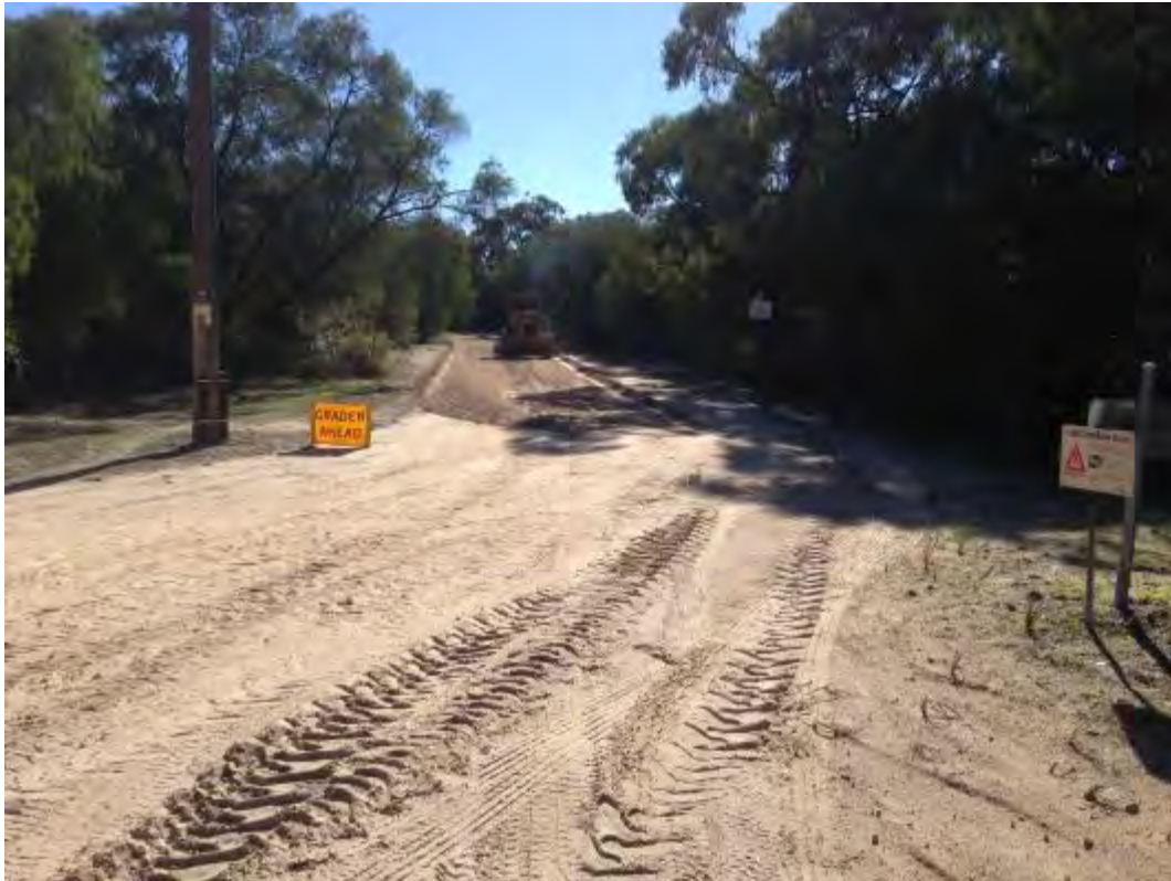
PBR North, SLK 0.05, unformed sandy track. Note power pole at edge.
