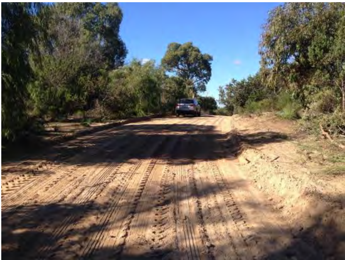
PBR North, SLK 4.8, poor sight distance on crest curve
