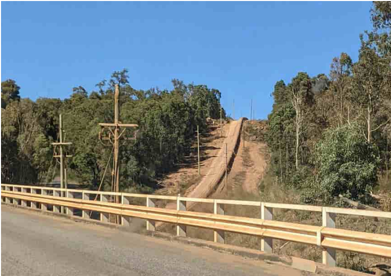
Photo 6-7 Example of existing conveyor for Myara Region
