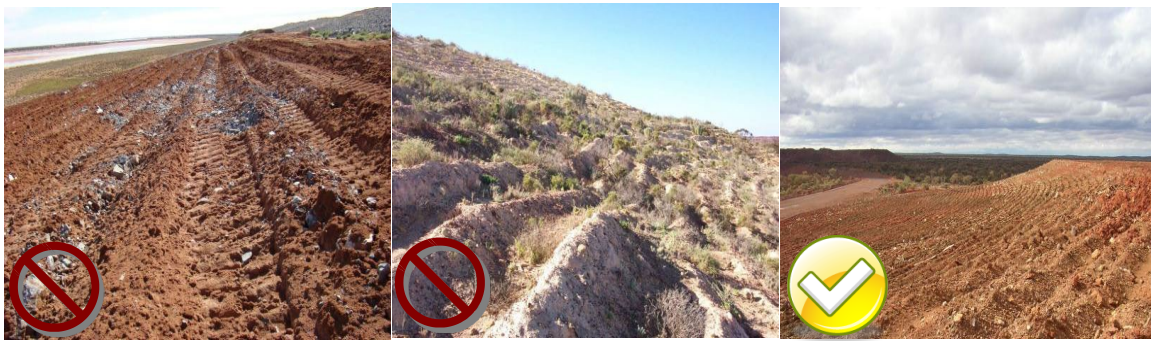
Figure 7: Example: (Left) single tine ripping leaving track marks over contour rip lines. (Centre) rip lines deviating from horizontal contours creating a zone of convergence, (right) satisfactory contour ripping along contour.
