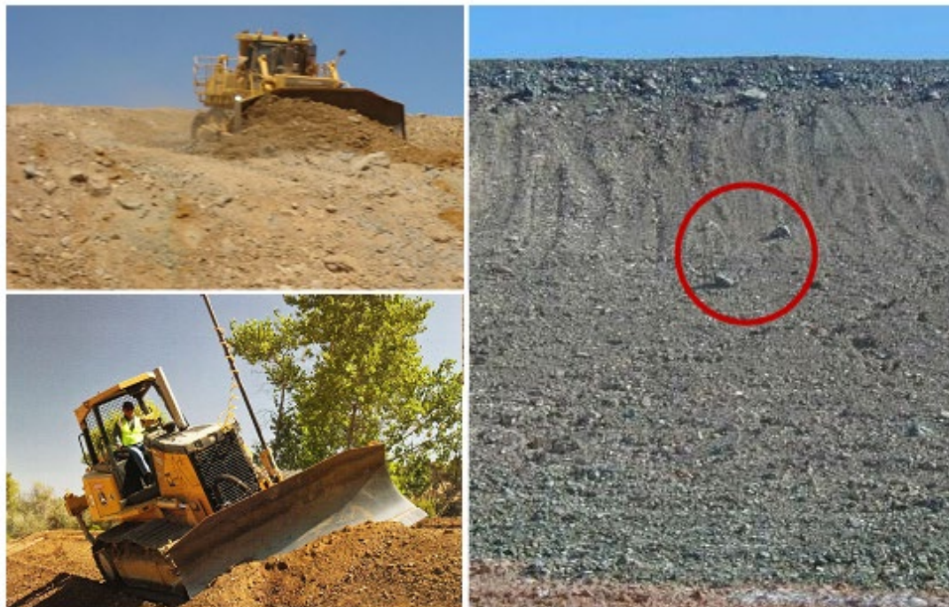
Figure 2: (Left Up) a dozer in the process of battering a slope. (Left Down) a dozer completing the final surface run by laterally traversing the battered angle. (Right) Example of converging features such as boulders and downslope track marks.
