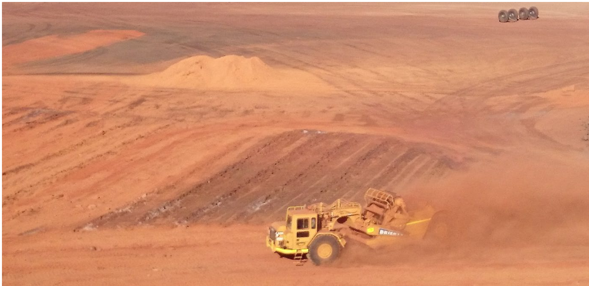
Figure 6: Scraper applying topsoil to a deep ripped hardstand area
