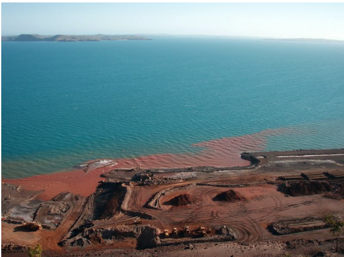
Figure 5. Plume from the Stage 3 seawall in windy conditions. Photo taken at 1615 29 August 2009.
