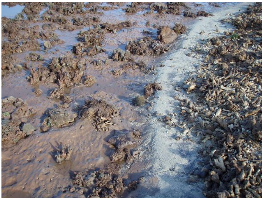
Figure 4. Boundary between the sediment-affected inner reef flat (left) and the section of reef flat uplifted by the seawall subsidence (right) in September 2009.
