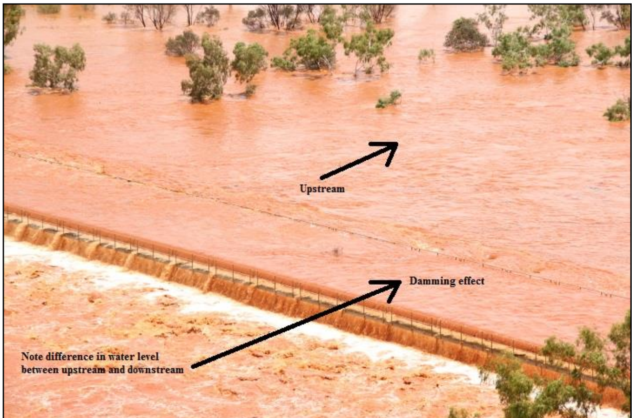
Figure B04 - Level difference across Rio Tinto Fortescue crossing railway floodway – 25 January 2013
