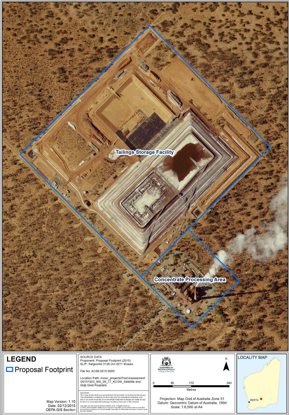
Figure 2: Location of proposal elements and disturbance boundary for the Gidji Gold Processing Plant
