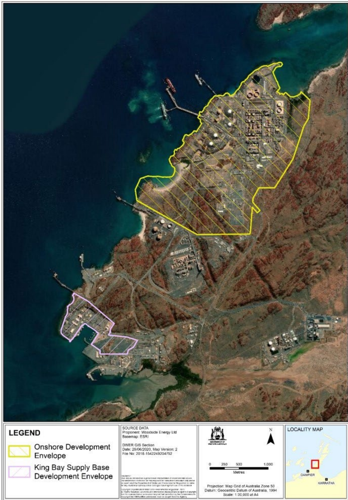
Figure 2: North West Shelf Project Extension Proposal onshore development envelope and King Bay Supply Base development envelope
