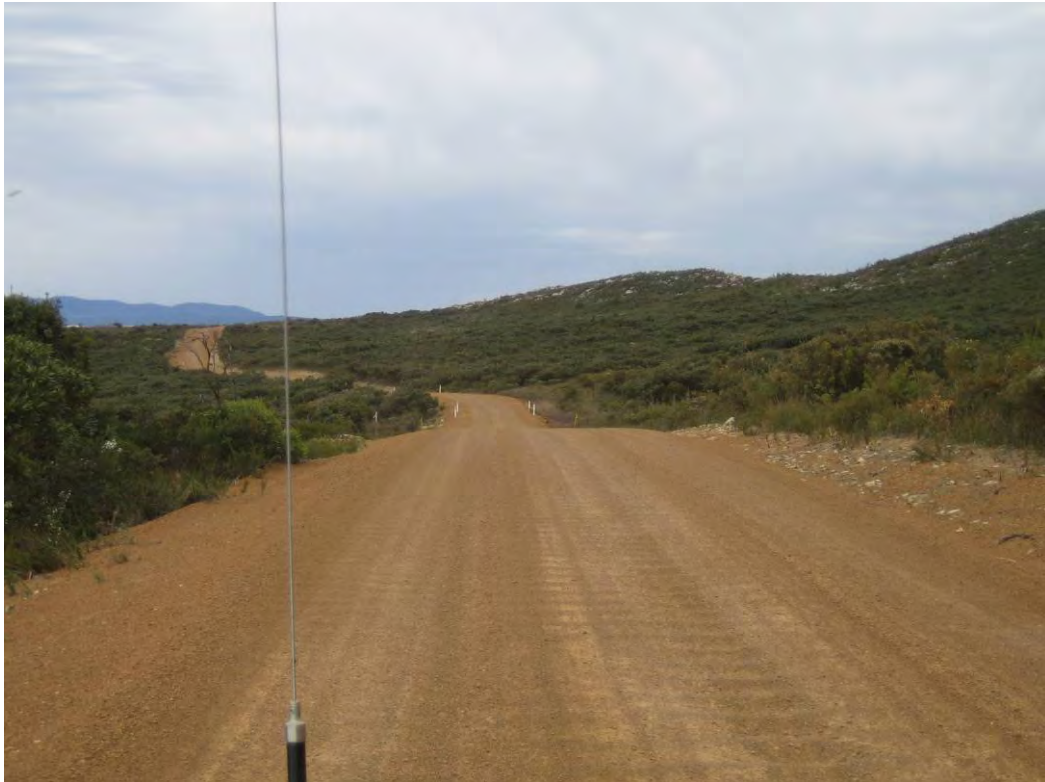
Figure 8 – Road cut into natural profile with some road batter slow to rehabilitate
