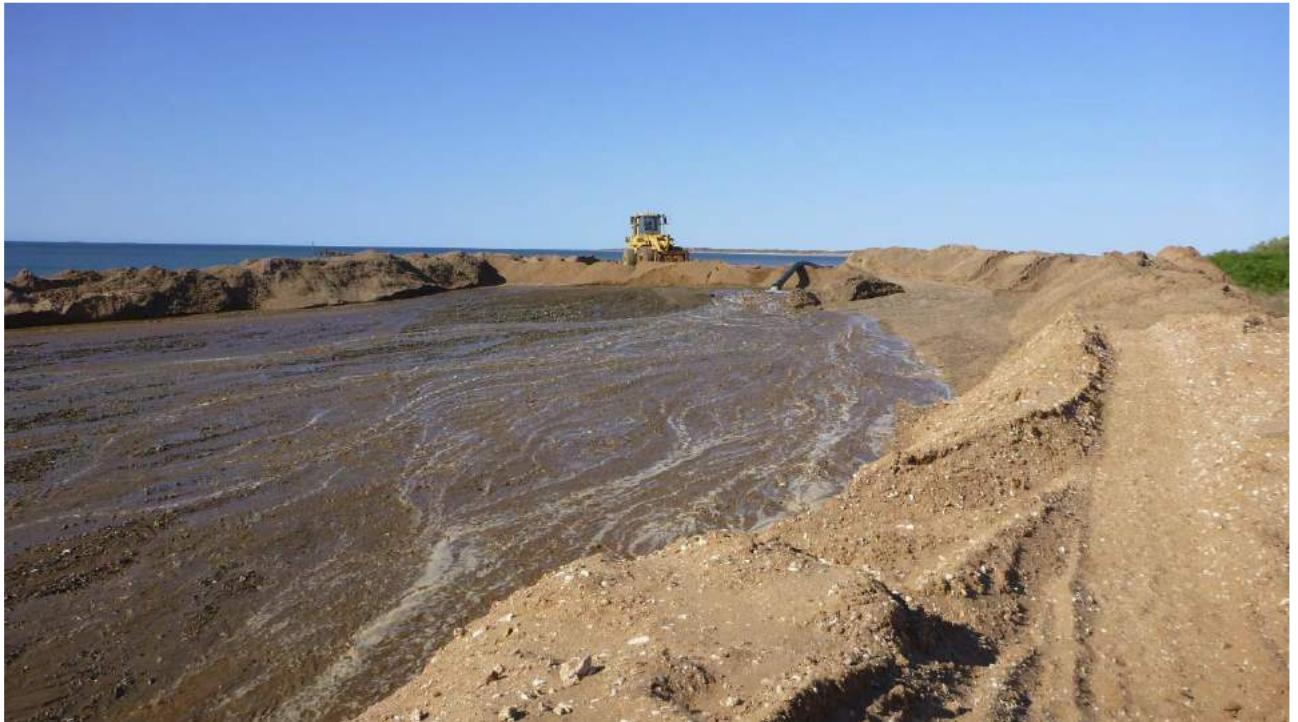
Plate 4-3 The beach being used as spoil disposal area for previous maintenance dredging of Beadon Creek (BMT JFA 2013)
