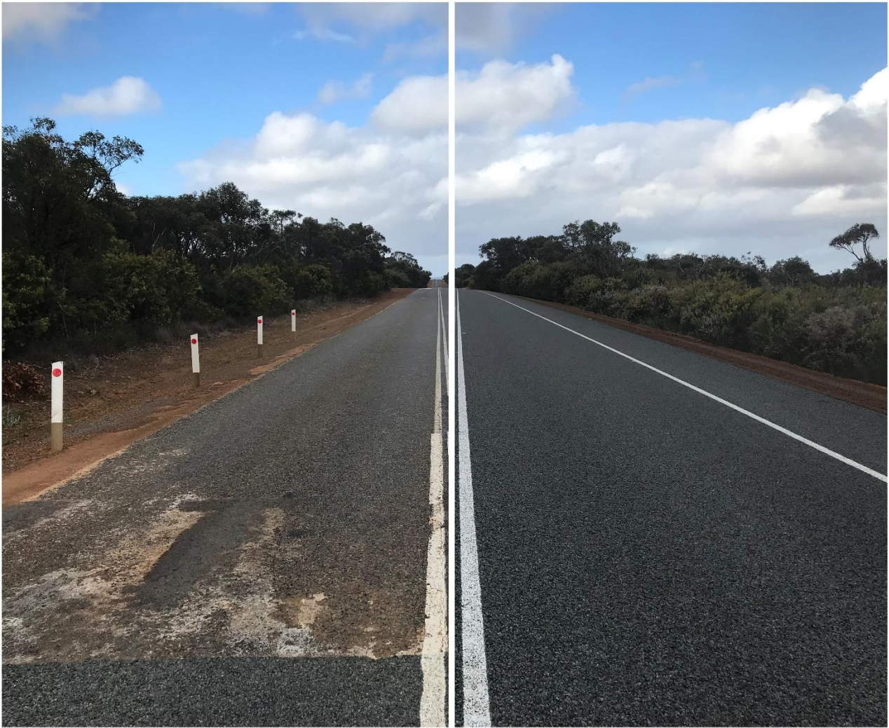
Figure 5 Before and After. Composite image of the existing South Coast Highway Kojaneerup Section (left image) and proposed road formation following works (right image (from previously reconstructed section)).
