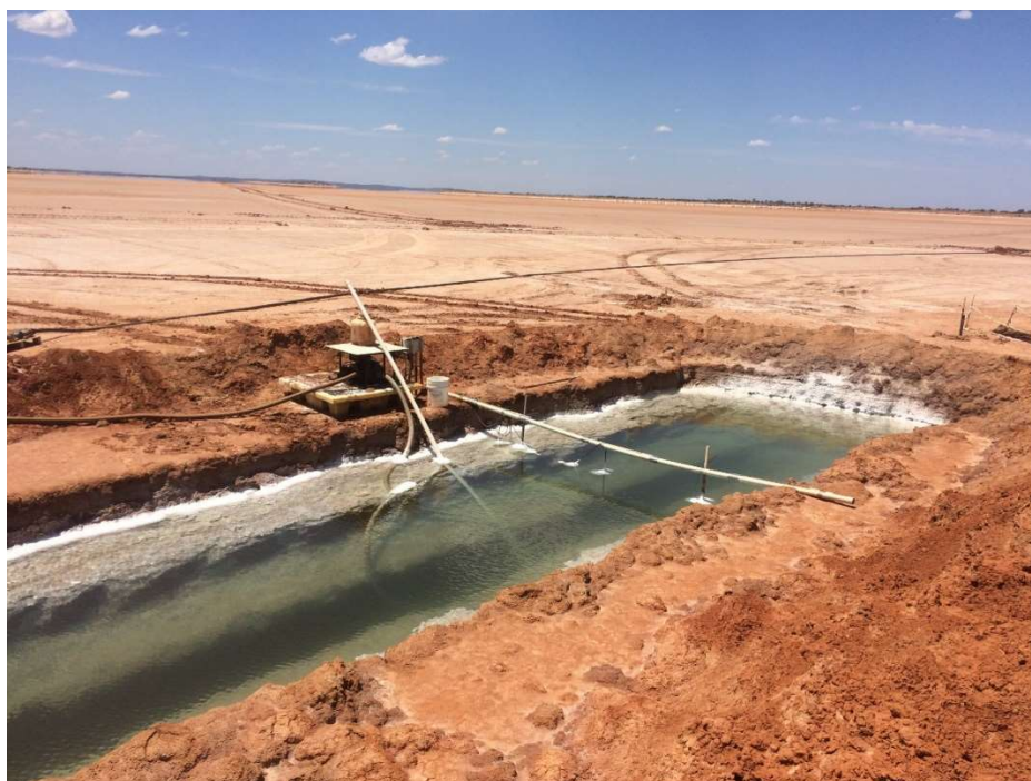
Figure 4.1: Trench and Pump Set-up
